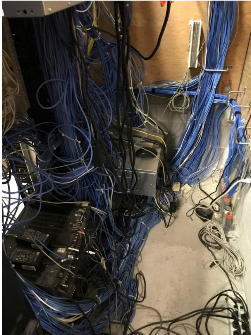
Figure 1 – floor area at back of racks in technology closet
